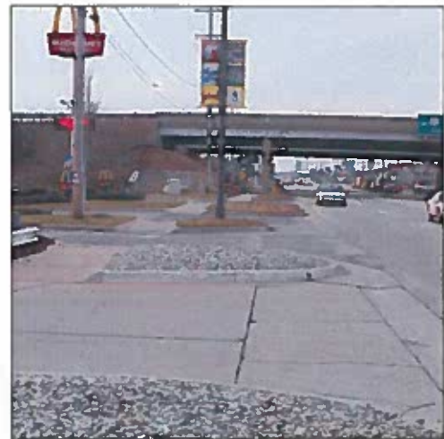
Multiple driveways on Pickard just east of US-127 lead to a variety of commercial uses.
